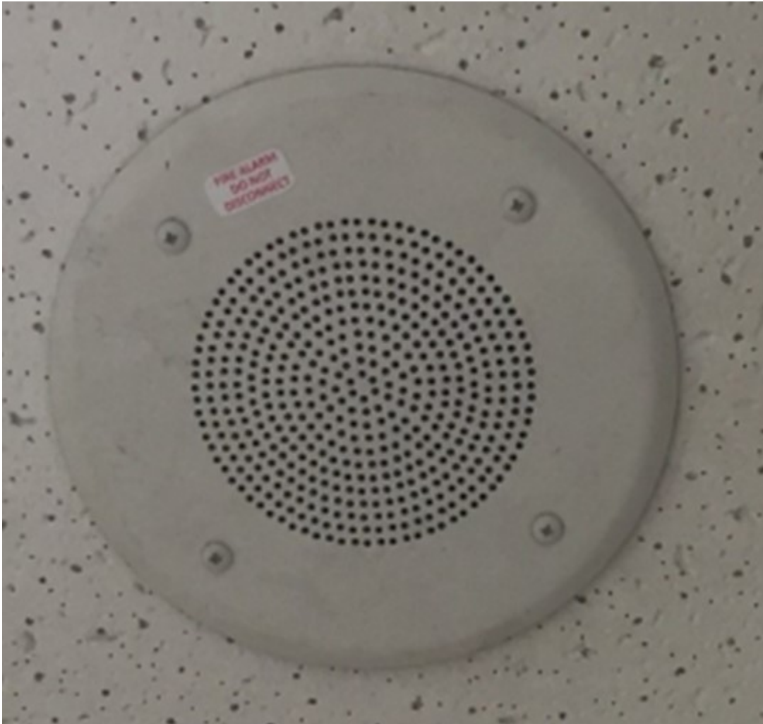
Figure 4-1: Typical Ceiling Loudspeaker with ECS Indicator
