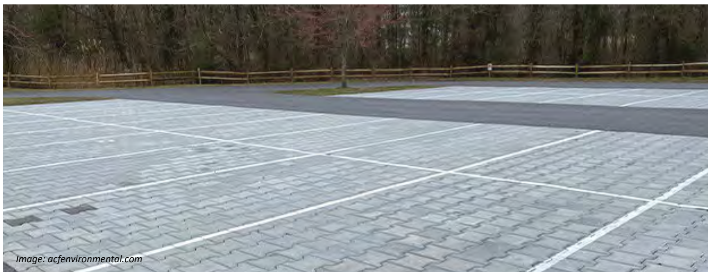
Articulated permeable paver mats at light vehicle parking can provide water quality and capture volume.
