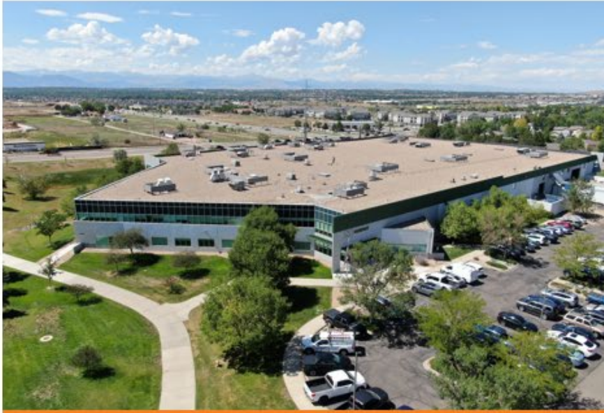
Colorado Central Office - Thornton, CO
