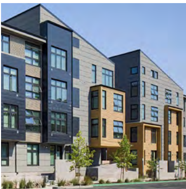
Fiber cement panels unexceptionable.
